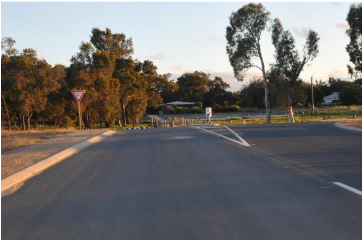
Finding 2.3 – Insufficient Approach Sight Distance on approach to intersection
